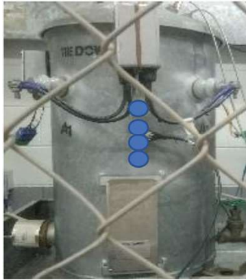
Figure 3 Test laboratory single-phase transformer
